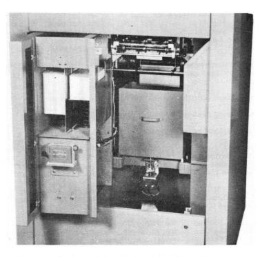
This view of the rear of the Card Sensing-Punching Unit with the rear panel open shows the Chip Pan as well as the Card Receivers.
